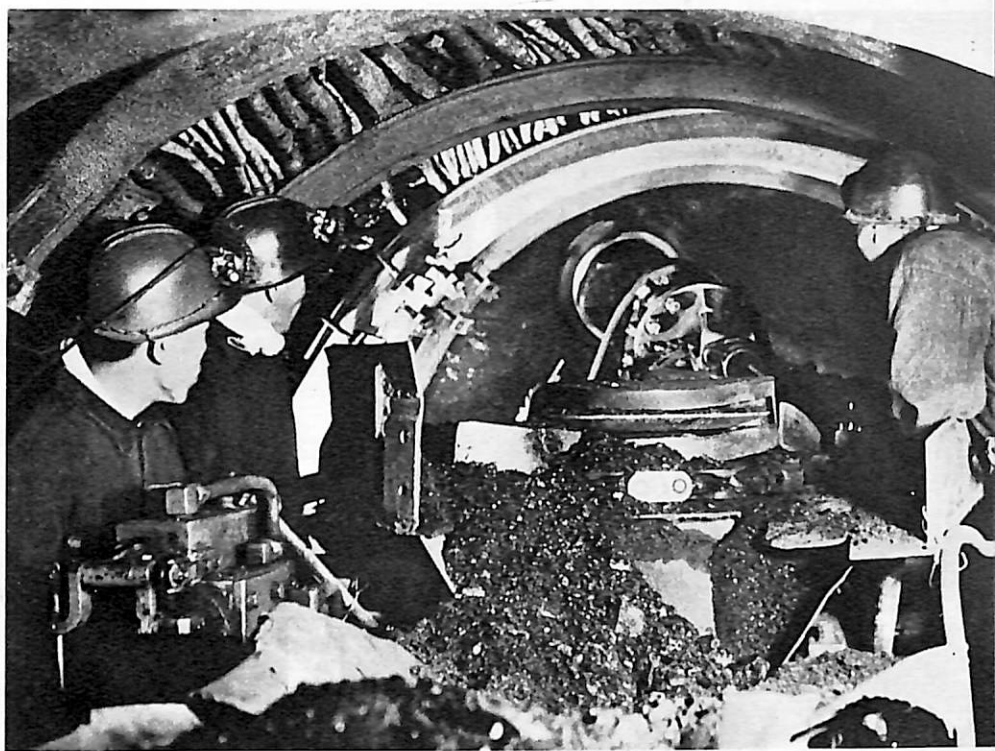
Kailuan miners in Hopei province tunneling with a cutting machine they made themselves.
